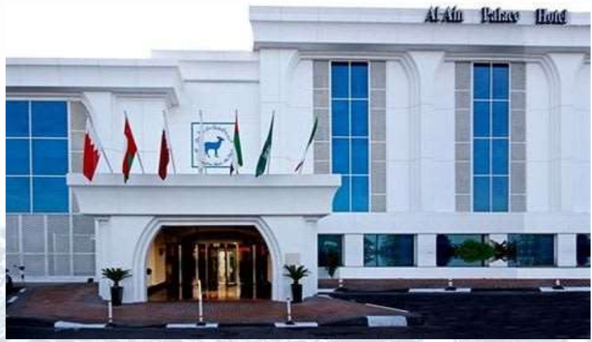
Al Ain Palace Hotel – Maintenance Works
