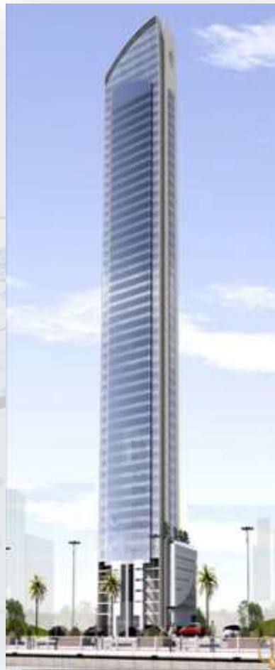
Sarayya Creek Abu Dhabi Tower 52 floors
